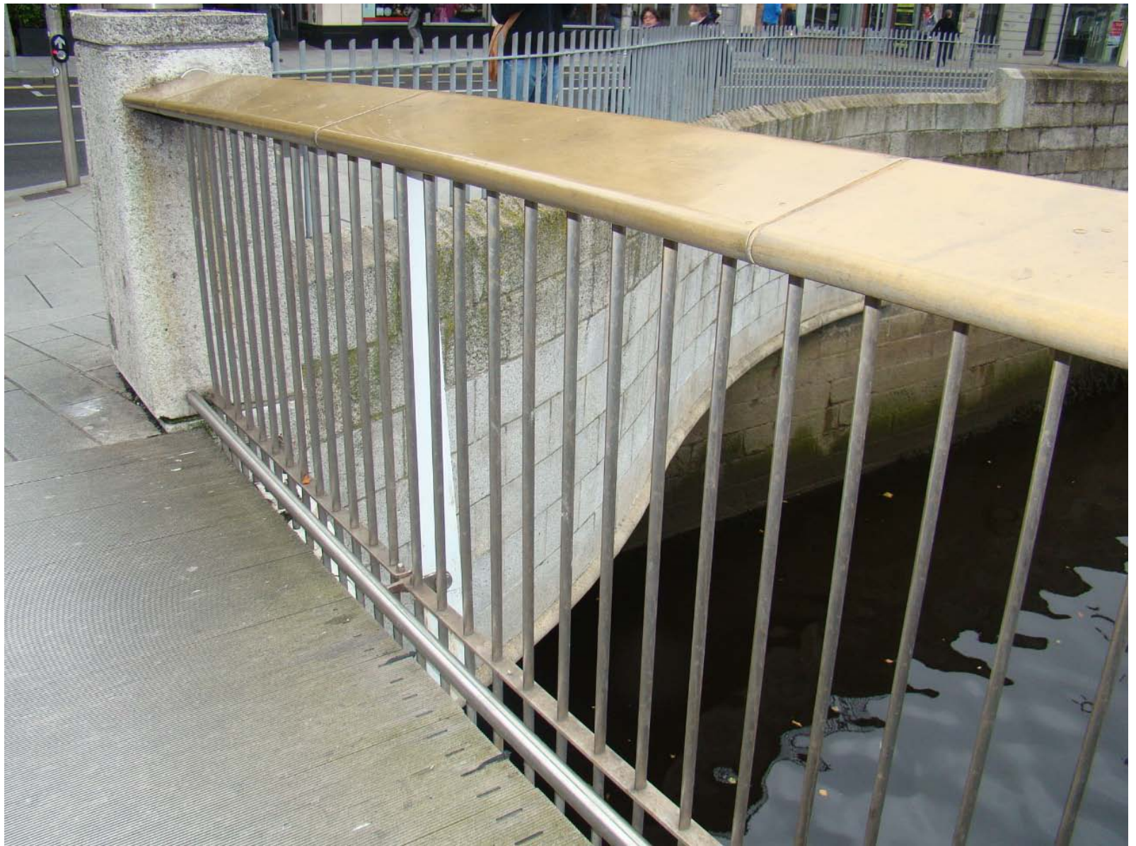
STAINLESS STEEL BALUSTRADE WITH A BRONZE ALUMINIUM HANDRAIL
