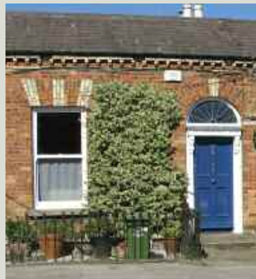
A typical brick-fronted, nineteenth-century house with solid masonry walls, single-glazed sash windows and slate roof
