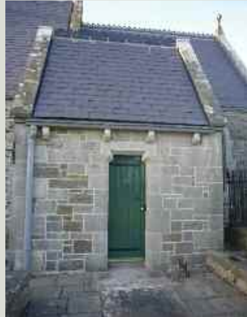
A special detail was used to deal with the small additional height that resulted from adding insulation to the roof build-up; stone blocks were added under the reinstated cast-iron gutter
