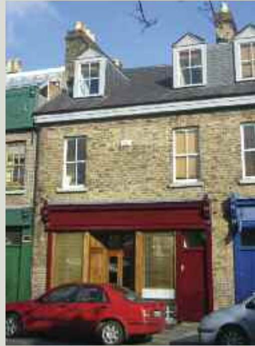
Although this traditionally built building is not a protected structure, it has been refurbished in accordance with best conservation practice
