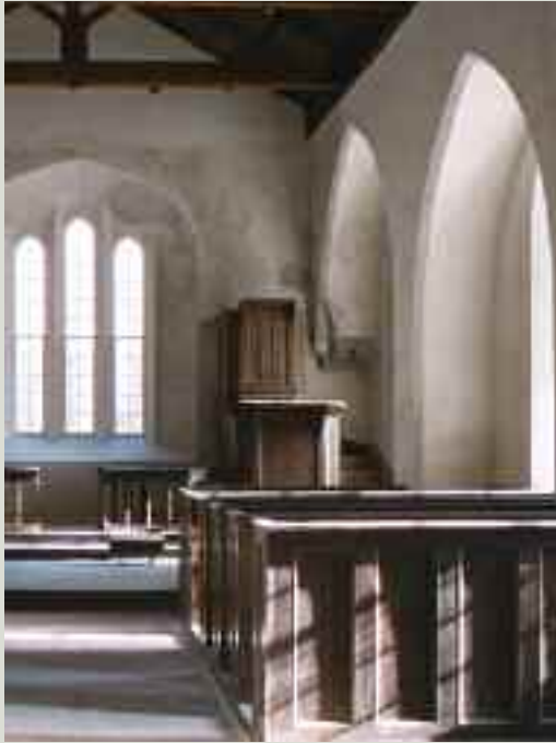
Box pews were the traditional way of keeping church-goers warm in an unheated, or poorly heated, church. The timber floor to each pew provided a warm surface underfoot, while the 'box' protected its occupants from draughts
