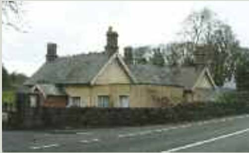
Cottages prior to refurbishment
