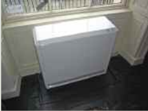
A storage heater fitted in a Georgian house. The low height of the storage heater allows for operation of the shutters at night and does not block the window
