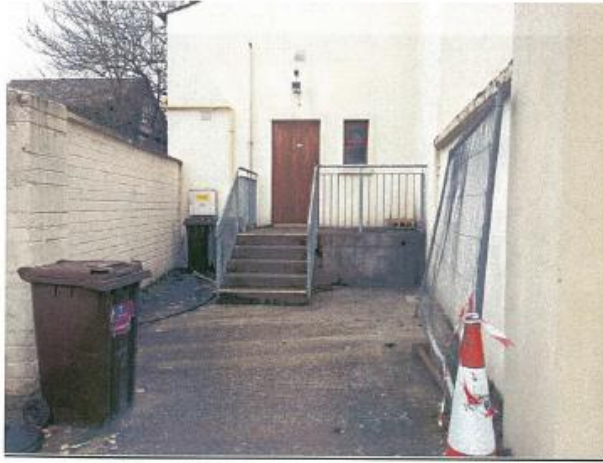
2. View of Service Yard adjoining West façade
