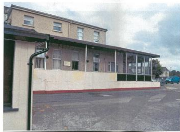
4. View from Horse Barrack Lane (South)
