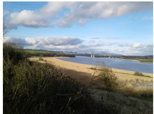
View from Carrickcloney of the route of the proposed Greenway to the New Ross By-Pass Bridge
