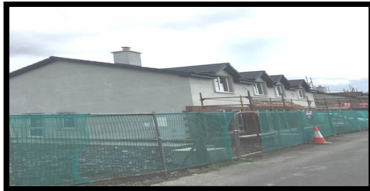
6 Units in Mooncoin (Chapel Street & New Street) under construction
