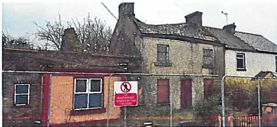
Site 2: Pair of derelict houses to be demolished & replaced
